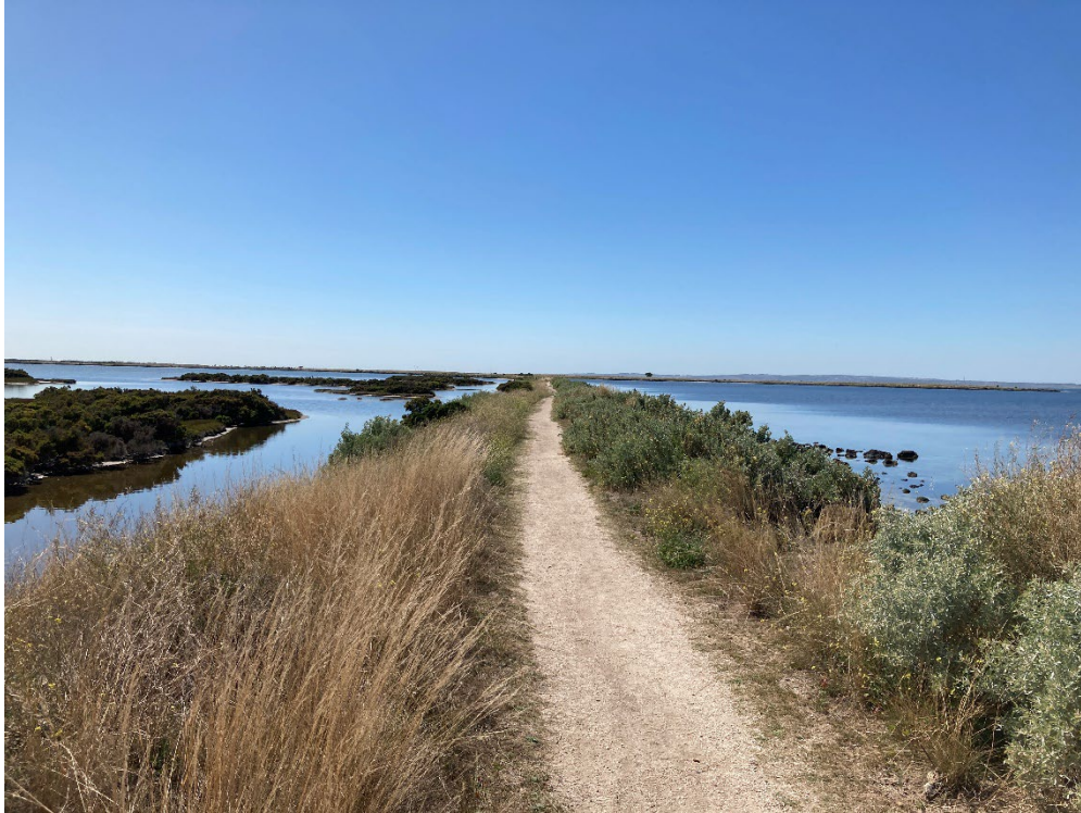
Plate 7 Walking track along Avalon Foreshore Road reserve with Port Phillip Bay on right and lagoon of the former Avalon Saltworks on right (February 2021)
