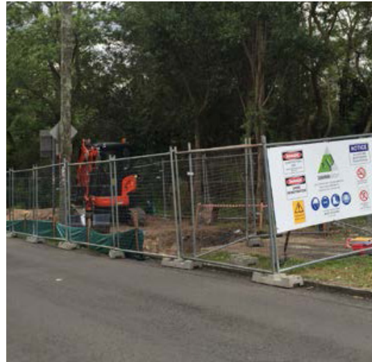
Maintenance and inspection activities on a section of a pipeline.
