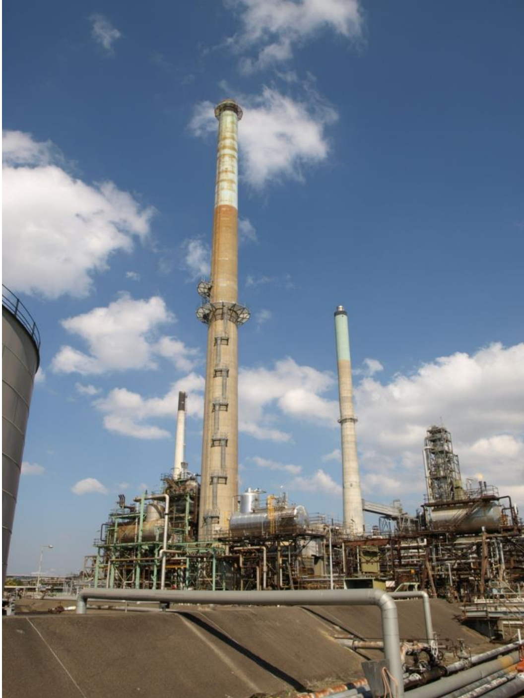
Plate 15 Boiler Stacks at the Project Area
