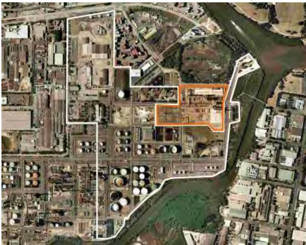
FIGURE 3.3: CLYDE TERMINAL LAYOUT SHOWING LYONDELL BASELL
