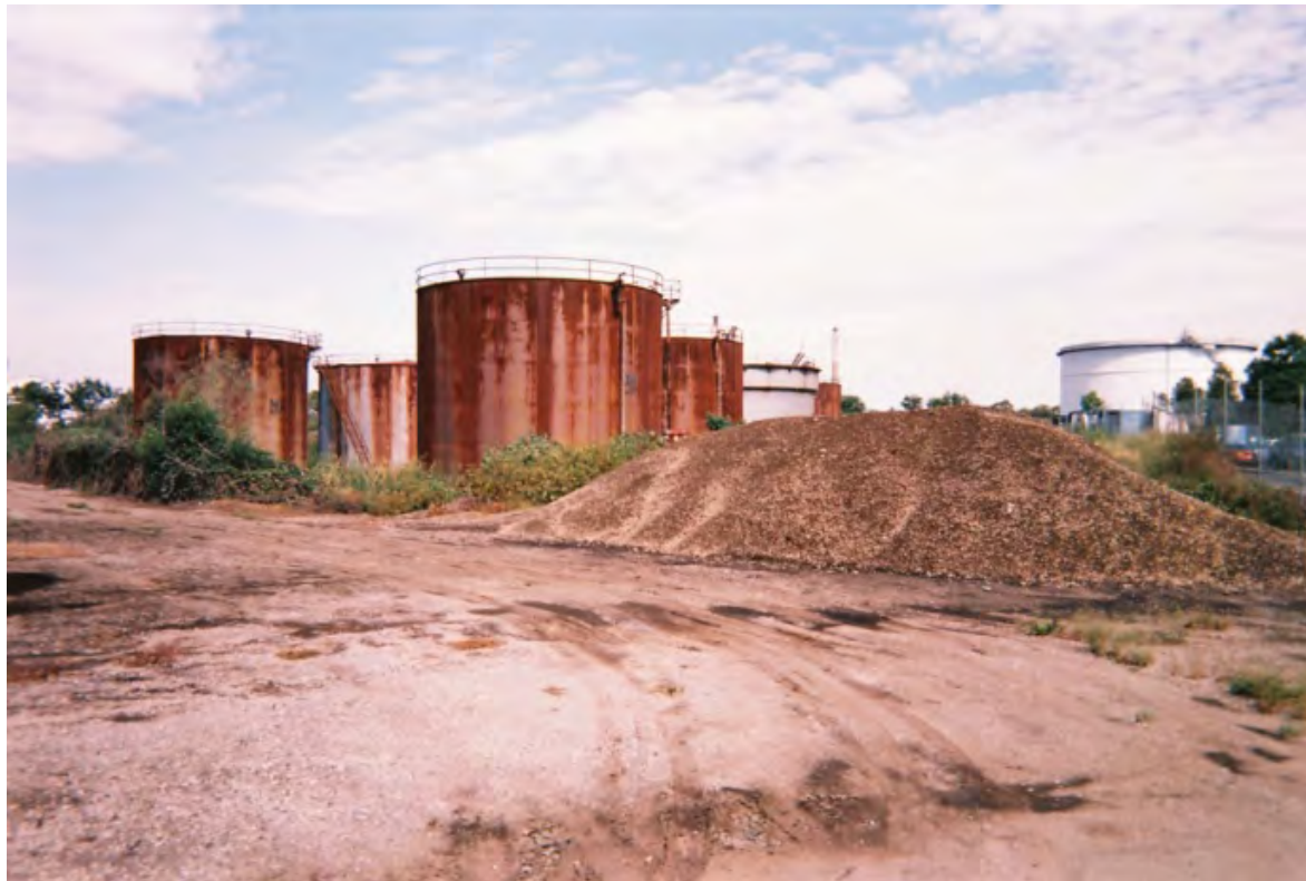
Plate 1 View of Mobile Tankfarm from the north, including neighbouring industrial properties
