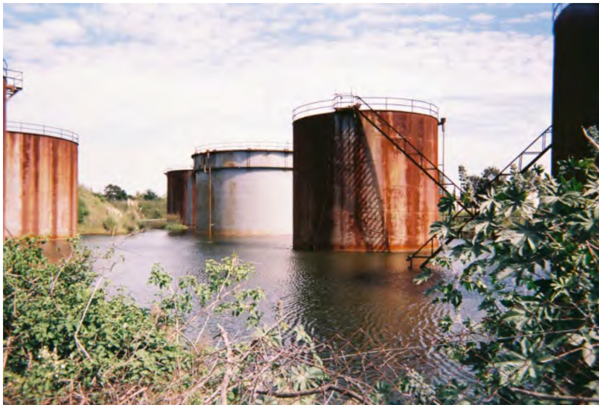
Plate 2 Mobil Tankfarm from the east
