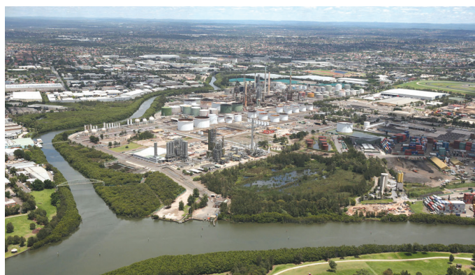
Aerial shot of Clyde Terminal, Parramatta
