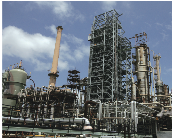
Some of the redundant equipment to be cleaned and demolished
